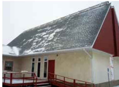
Roofing shingles, St. James the Apostle Church, Thompson, MB
